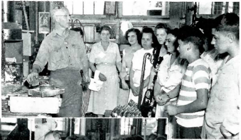
Ralph Adams amazed visitors with his dexterity in handling molten lead as he showed how joints were wiped by hand.
