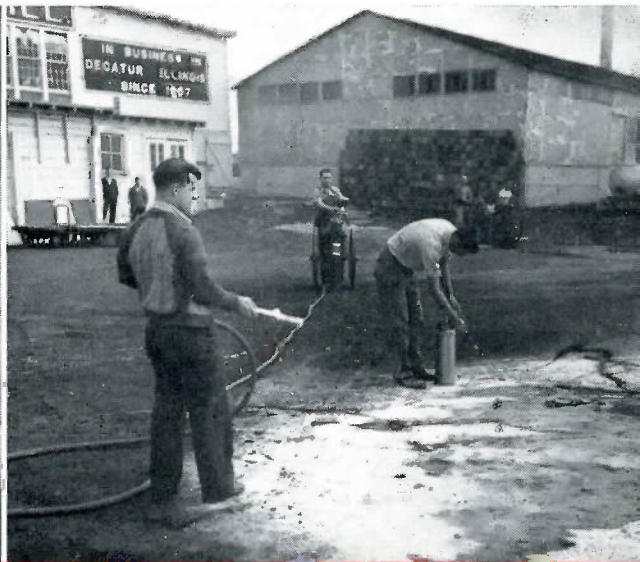
George Lebo, milling machine operator, uses a carbon tetrachloride hand extinguisher to put out the last traces of the blaze while Sulwer stands by.
