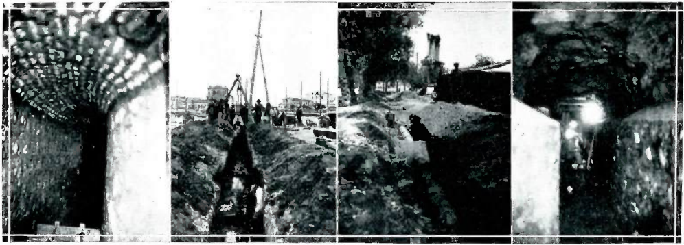
Reading from Left to Right—Interior view of repaired and enlarged section of ancient Hadrian Aqueduct. The section of the old aqueduct may be seen at bottom of picture.
