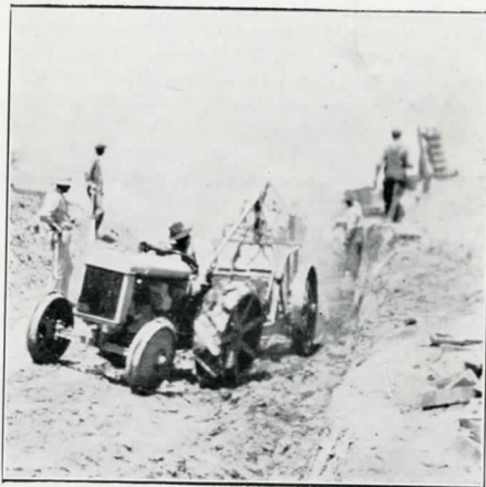
Tractor grading at Plant 9
