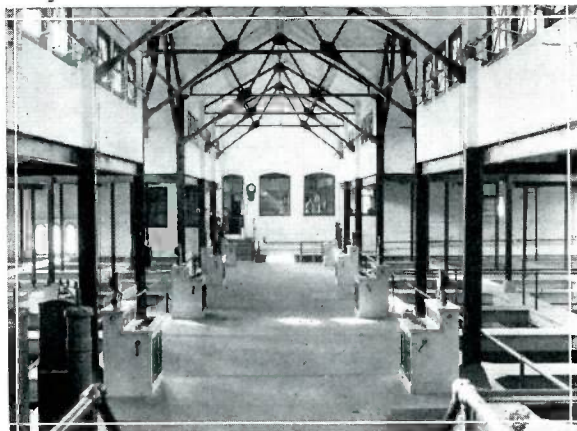
A portion of the filter gallery at Grand Rapids showing eight of the twenty filters.
