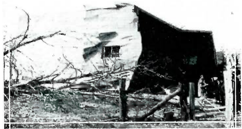
An elevator at Buffalo Hart wrecked by the cyclone of April 23. The building, about fifty feet high, was lopped over on its side. The elevator fell to the south while all other buildings fell to the north.
