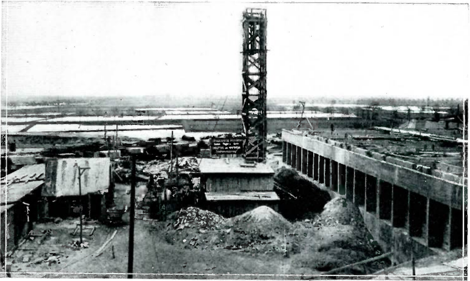
View of the marsh gas works at Berlin which makes gas, not from coal, but from irrigation and water waste of the town, thus proving a new and economical device. —Photo by Underwood & Underwood.
