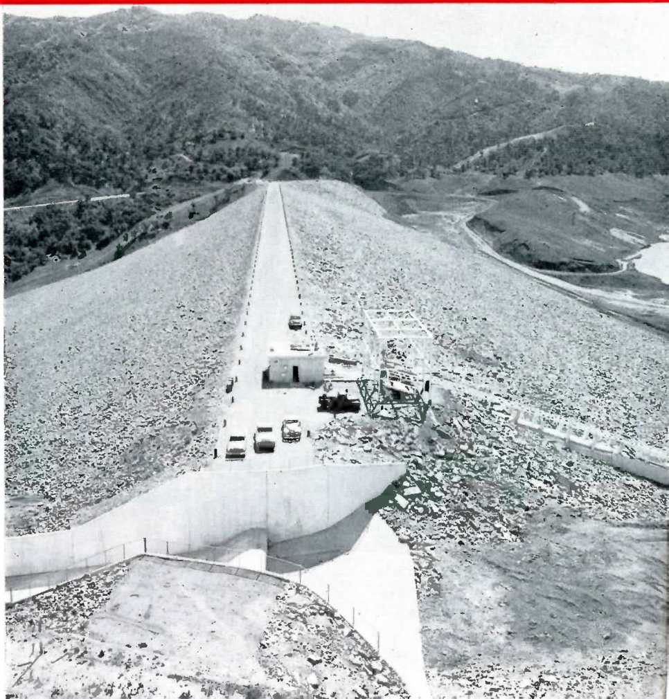
The 285-foot high dam embankment, outlet works, intake structure and spillway inlet in the foreground are viewed from atop the left abutment. The crest length of the dam is 2,060 feet and goes from a base width of 1,625 feet to a crest width of 40 feet.
