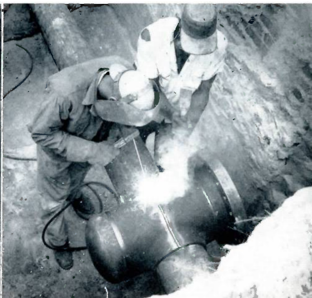
Below left, the welding control fitting is in place. C. V. Brooks is the welder and Calvin Slade is the helper. At right, the welding control fitting halves are on the gas main. The welder is Robert Brown, the contractor's employee, and L. C. Range.
