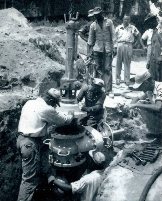
At left, workmen place the Mueller machine with cutter on the control valve to begin cut. Left to right in ditch, L. C. Range, Chester Campbell and Marion Boyce. Standing from left, Paul Dooley, Calvin Slade, H. W. Cessna, A. H. Abernathy and J. H. Lookey. In the photo at right, the 10" Mueller fitting is shown welded in cutting position with the control valve. The pipe cutting machine shown on this main will be used to cut the main in two after cut is made and rubber stopper is inserted in Mueller fitting.
