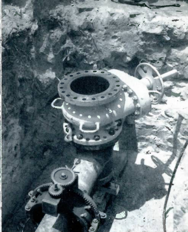
At left, workmen place the Mueller machine with cutter on the control valve to begin cut. Left to right in ditch, L. C. Range, Chester Campbell and Marion Boyce. Standing from left, Paul Dooley, Calvin Slade, H. W. Cessna, A. H. Abernathy and J. H. Lookey. In the photo at right, the 10" Mueller fitting is shown welded in cutting position with the control valve. The pipe cutting machine shown on this main will be used to cut the main in two after cut is made and rubber stopper is inserted in Mueller fitting.
