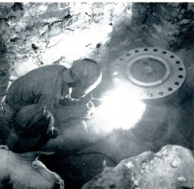
Below left, the welding control fitting is in place. C. V. Brooks is the welder and Calvin Slade is the helper. At right, the welding control fitting halves are on the gas main. The welder is Robert Brown, the contractor's employee, and L. C. Range.
