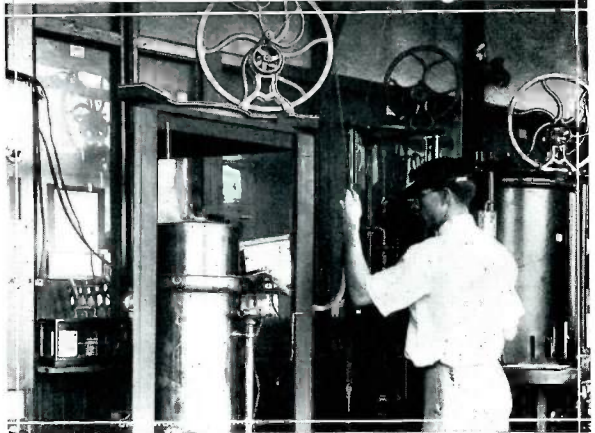
This is a picture of H. S. Bean of the gas measurements instruments section of the U. S. Bureau of Standards in Washington, testing a portable cubic foot standard by comparison with the Bureau's standard cubic foot bottle.
