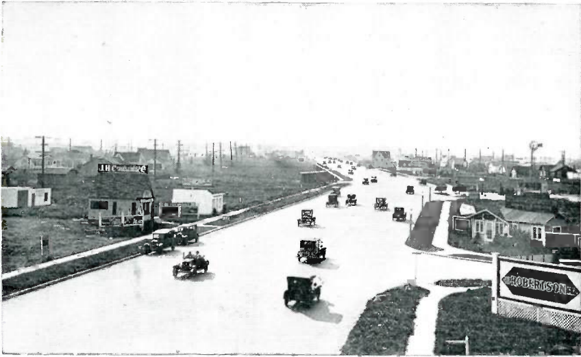
Pico Boulevard from Los Angeles to the ocean with more than 10 miles of 73 feet wide concrete 8 inches thick. This boulevard provides for four lanes of traffic each way.
