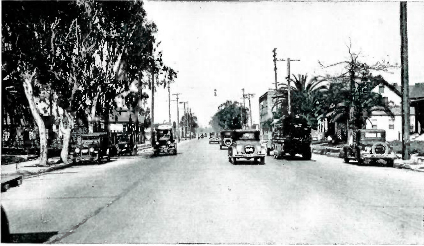
Washington Boulevard, between Central and Alameda, built in 1925 of 8 inch concrete. Carries extra heavy traffic but the wear has been negligible.
