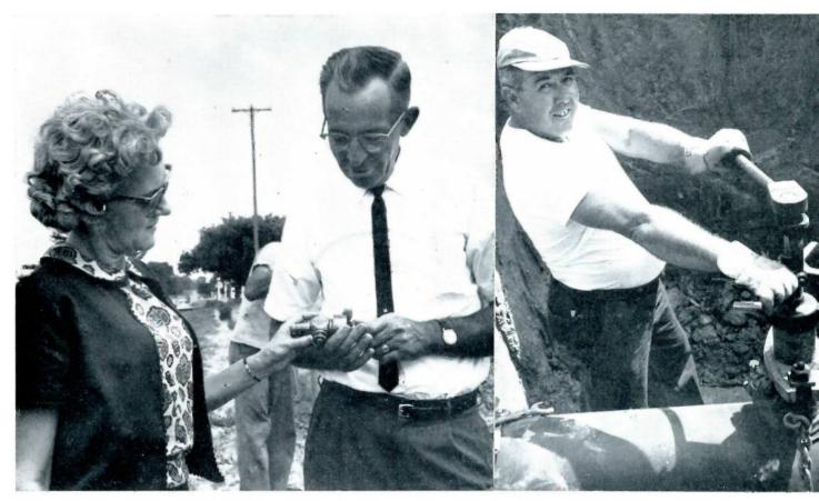
Lester Thornton, Water Superintendent, explains to Mayor Dunlap how the Mueller B-100 drilling and tapping machine (right) inserts a Mueller corporation stop into a main under pressure.
