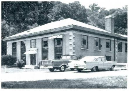
The original Griffey Lake Treatment Plant (above) has a filtration capacity of three million gallons daily. To meet increased demands for water, a large addition was started in 1954, providing total facilities which are capable of treating  $7\frac{1}{2}$  million gallons daily.
