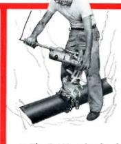
■ Fast, dependable service connections can be made on thin-walled pipe under pressure without interruption of service. ■ The special compression joint on the Mueller corporation stop provides a pressure-tight seal, while the short inlet threads assure a strong mechanical connection to the main.
