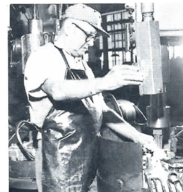
Eddie Theriault, a Mueller man for 30 years, skillfully operates a drill press which performs rough and finish reams on iron valve bodies. Reamers are produced in Sarnia by the tool room.
